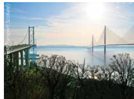
Forth Replacement Crossing achieved an overall 'Excellent' CEEQUAL rating with a score of 92.7%
